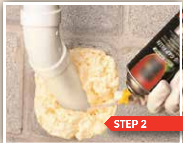
Step 2: Spray foam into steel wool.
