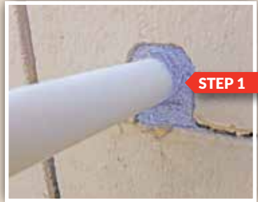
Step 1: Fill gap with coarse steel wool.
