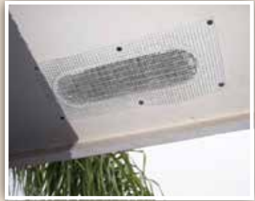
Soffit vent hole sealed with screen.*
