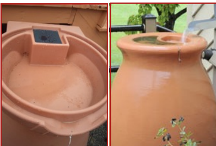
Modified or decorative tops will hold enough water to breed mosquitoes
