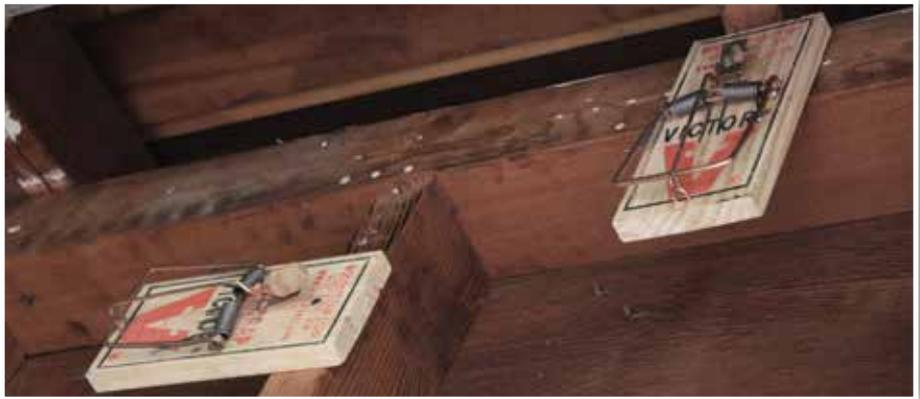
*Proper trap placement on beams and rafters. Note rub marks on beams indicating rat trails.*
