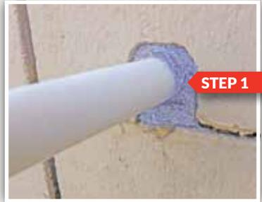
*Step 1: Fill gap with coarse steel wool.*
