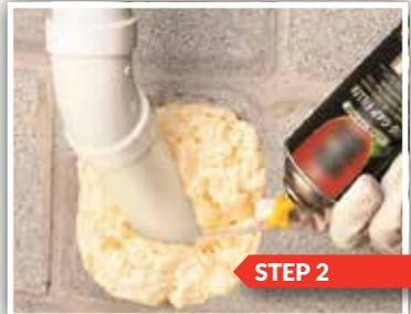
*Step 2: Spray foam into steel wool.*
